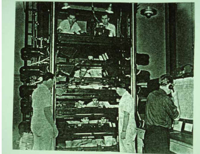
Figure 2a: Walt Disney's multiplane camera stand
